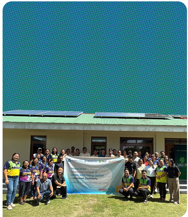
▲ INSTALLATION OF a 20 kWp solar energy system powering key public facilities, including Manamoc National High School, the community gymnasium, and the local health center.
