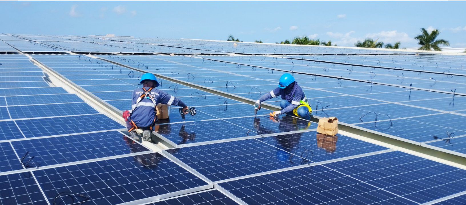
Installation of PV panels for the Kinpo Project in Lima, Batangas.
